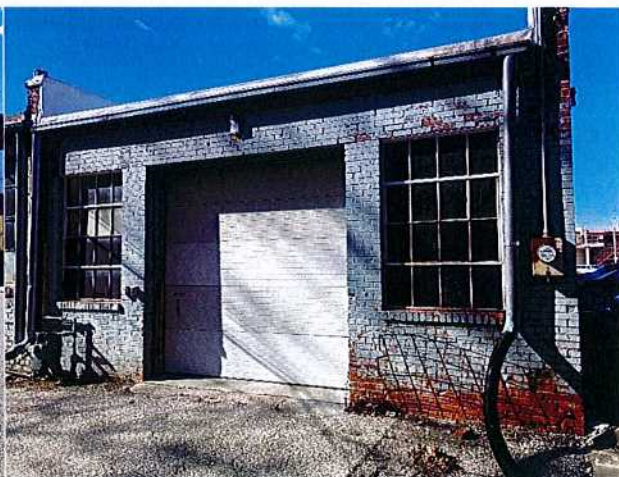
622 Mechanic east (alley) side of the building
