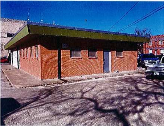
East side of the building.
