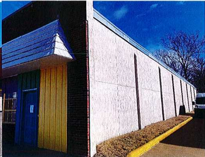
South side of the building
