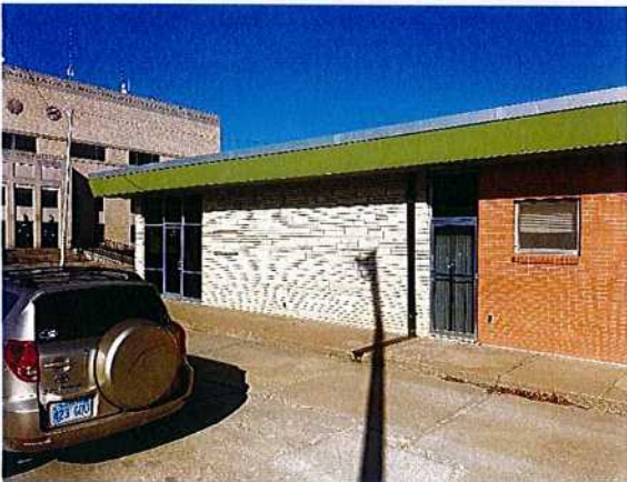
South side of the building.
