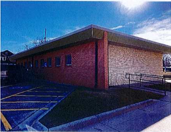
North side of the building.
