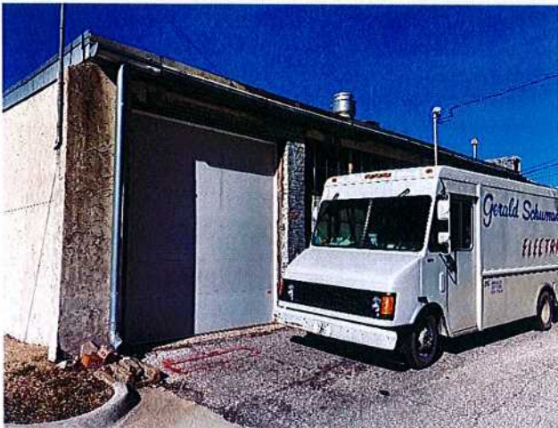
618 Mechanic east (alley) side of the building
