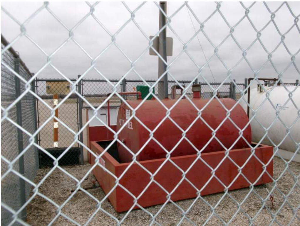
Existing MoGas Tank
