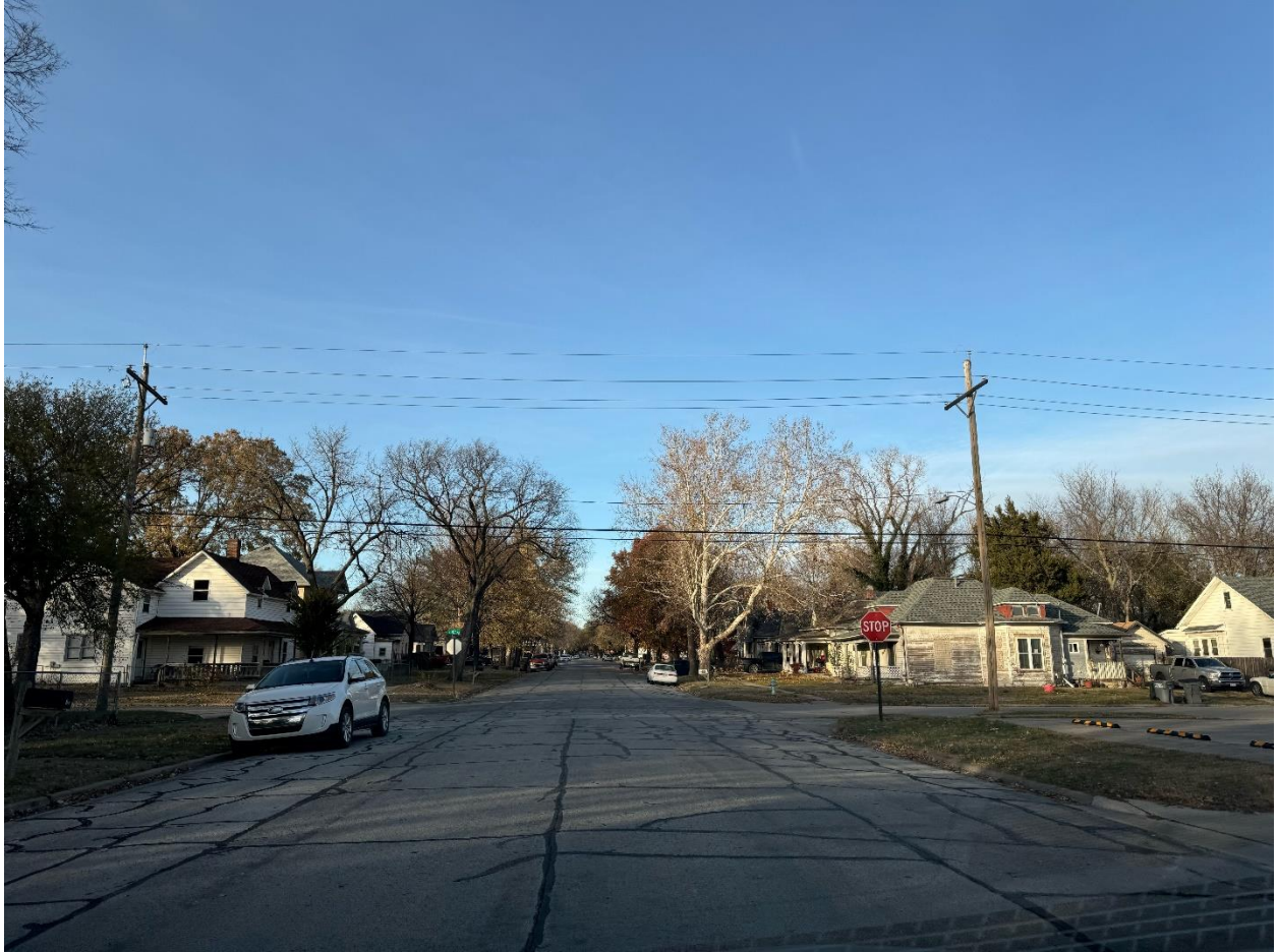
Neosho Street, near 4 th Ave. (looking north), existing asphalt over brick
