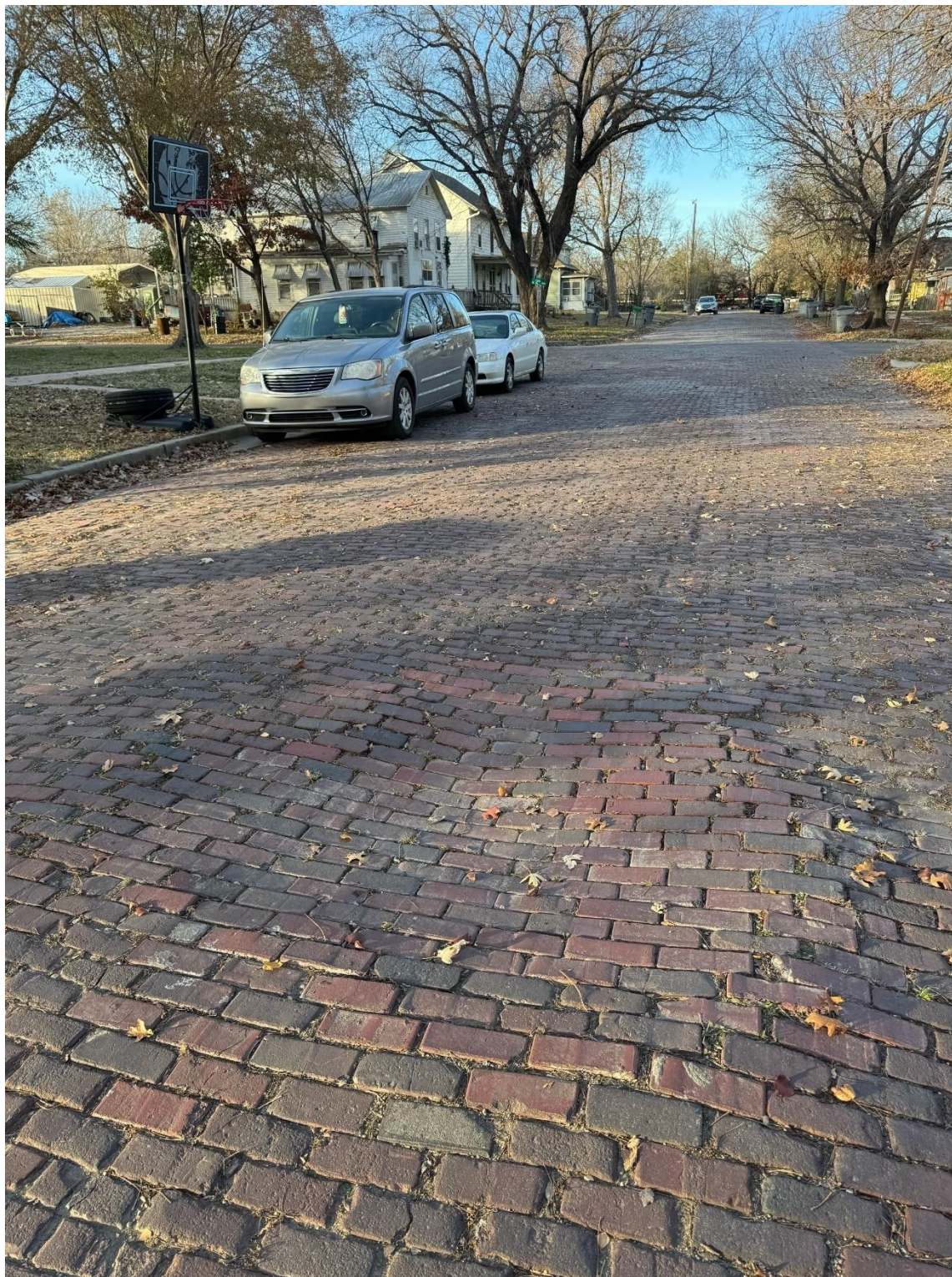
Neosho Street, about midway between South Ave and 1 st Ave (looking north toward BNSF)
