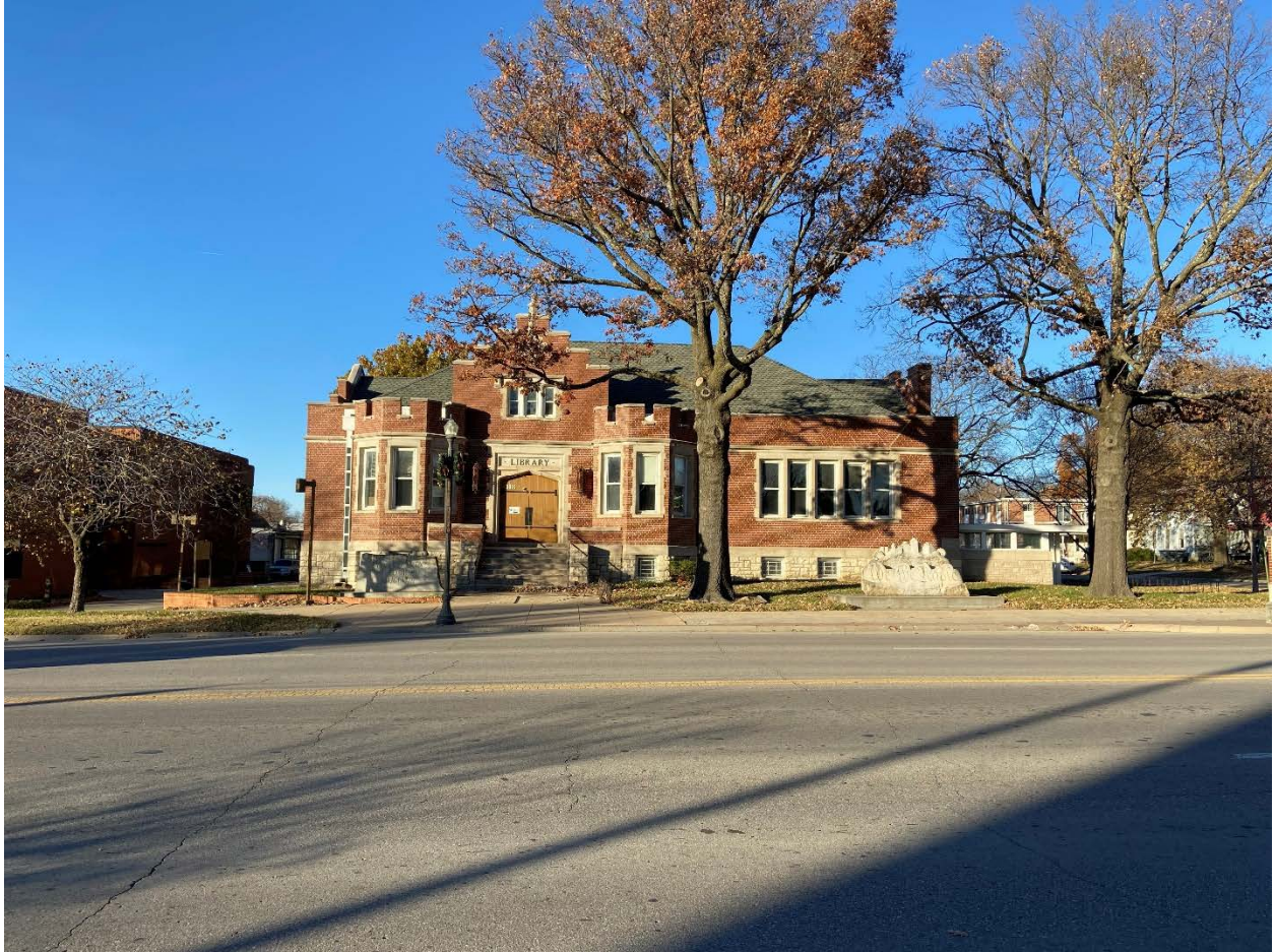
ABOVE South façade, main façade facing 6 th Street
