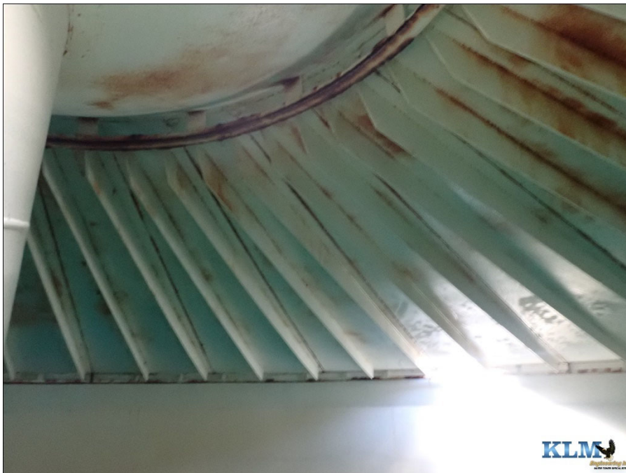
Photo No. 6 Overall condition of roof
