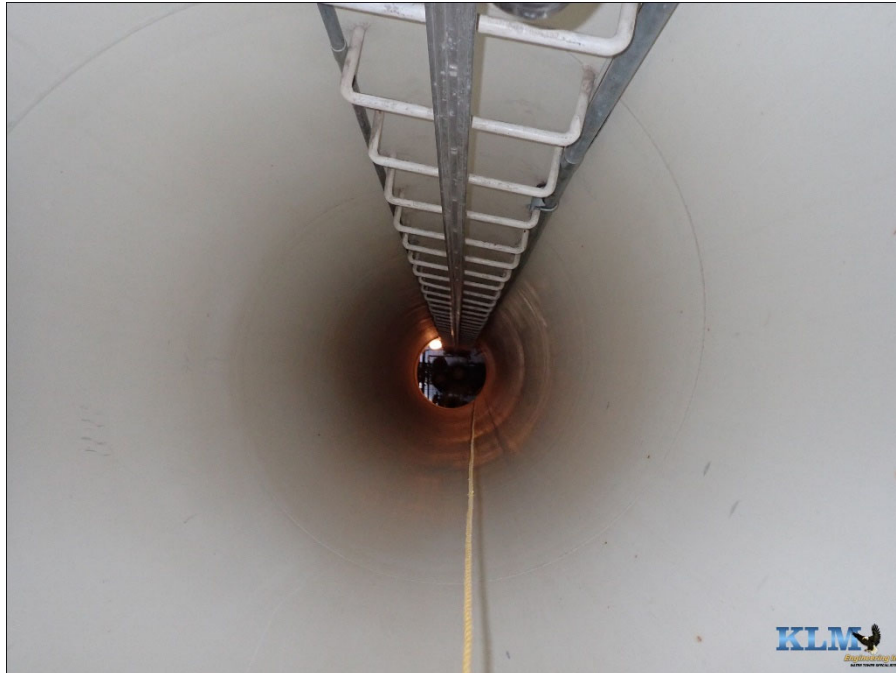
Photo No. 31 Overall conditions in drywell tube
