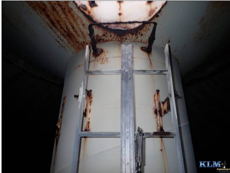
Photo No. 9 Wet ladder and top of drywell tube
