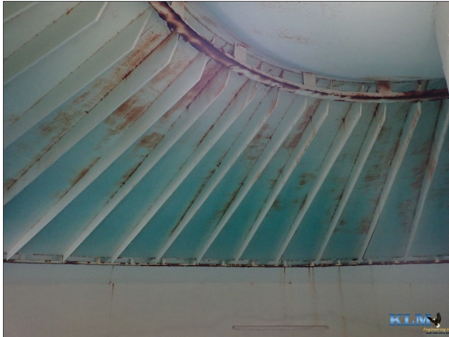
Photo No. 7 Overall condition of roof
