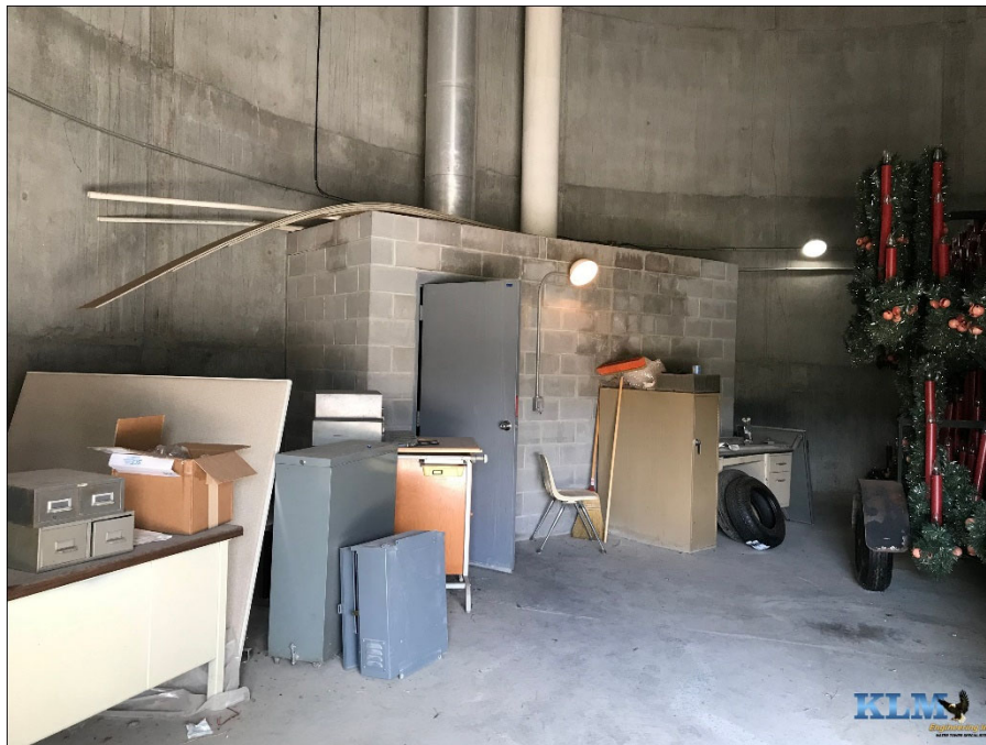
Photo No. 40 Conditions in tower base
