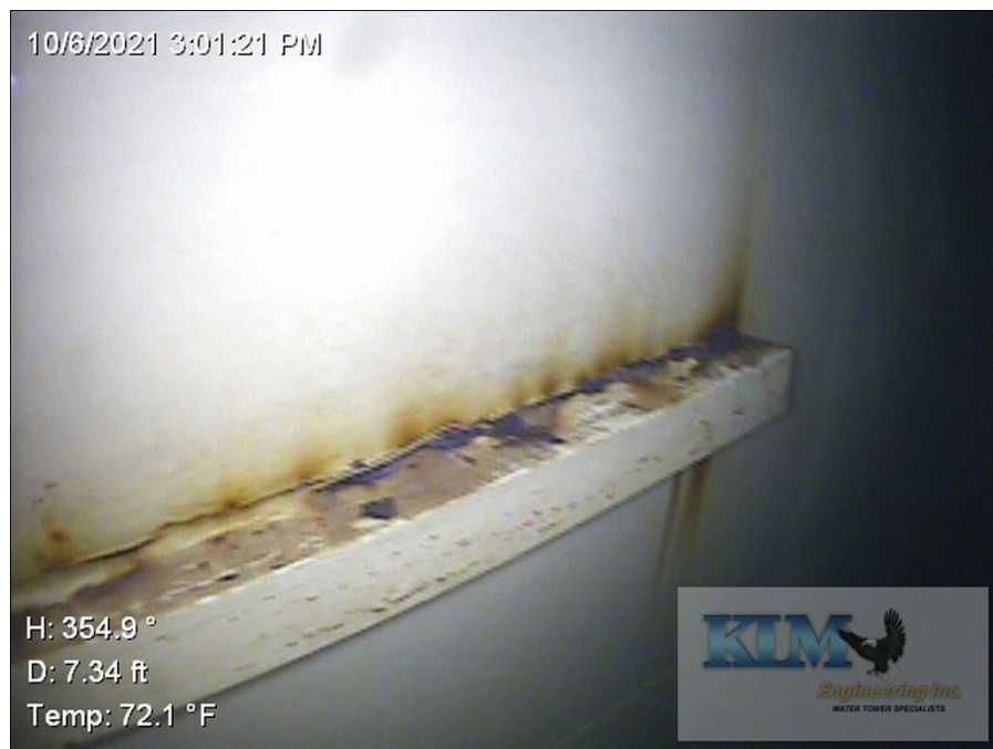
Photo No. 24 Condition of shell erection angles
