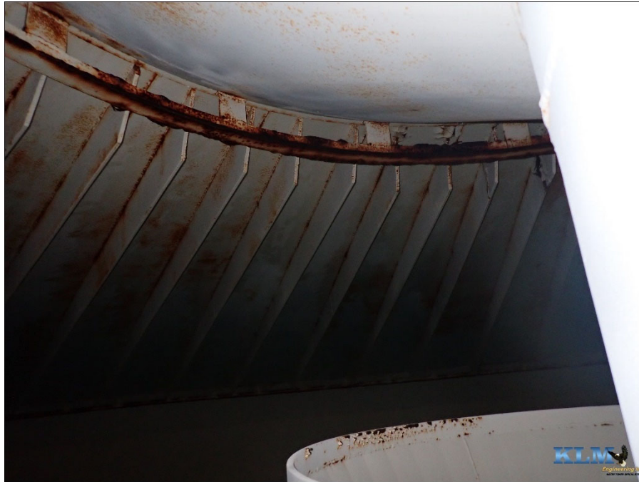
Photo No. 11 Inner T-rail
