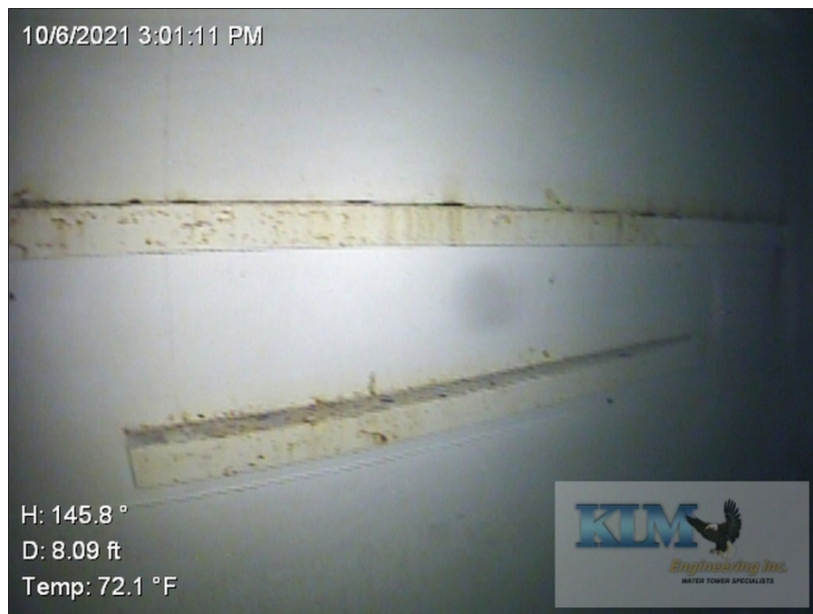
Photo No. 26 Shell erection angles
