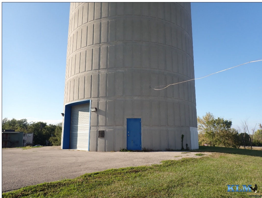
Photo No. 56 Base access
