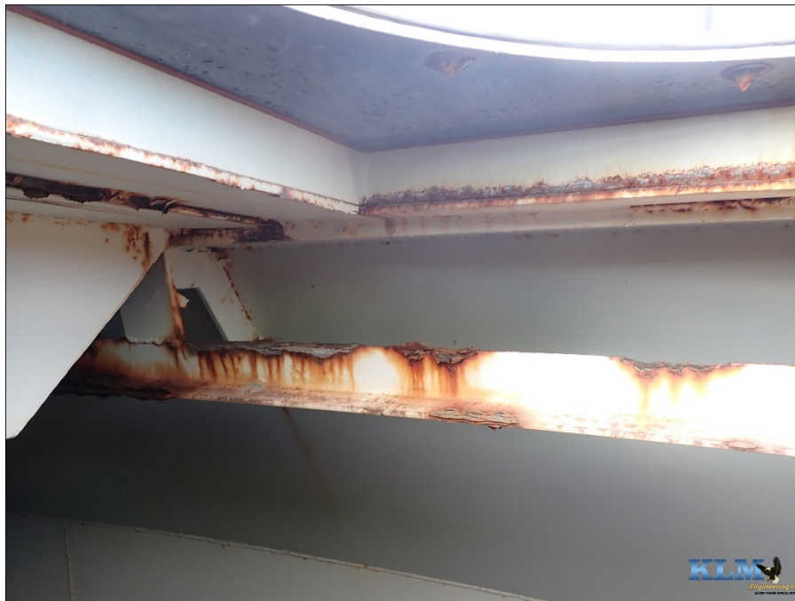
Photo No. 2 Outer T-rail and roof conditions
