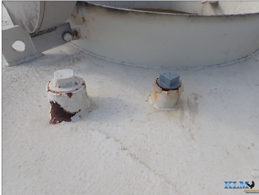
Photo No. 51 Roof couplings
