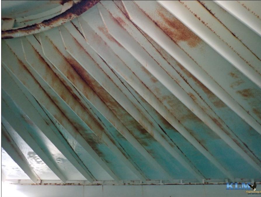
Photo No. 5 Overall condition of roof
