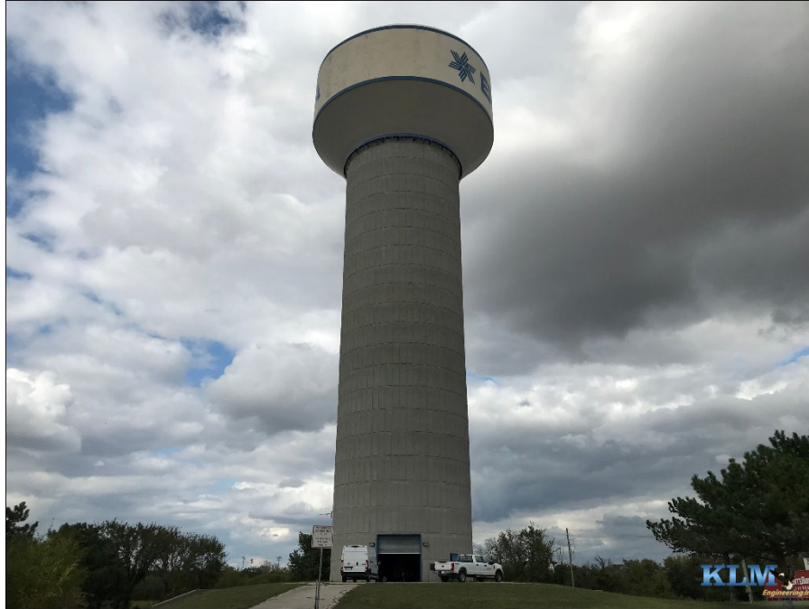
Photo No. 1 Overall view of the tower
