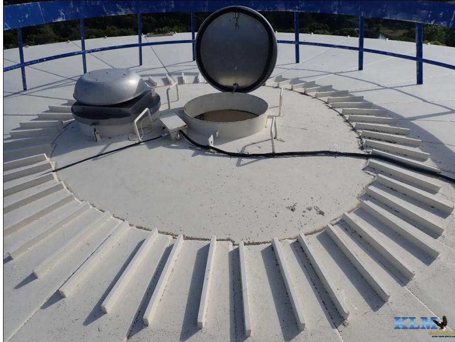
Photo No. 43 Overall roof conditions
