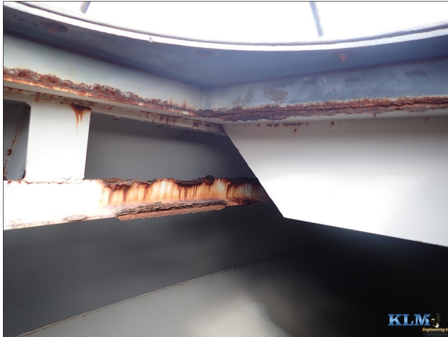
Photo No. 3 Outer T-rail and roof conditions
