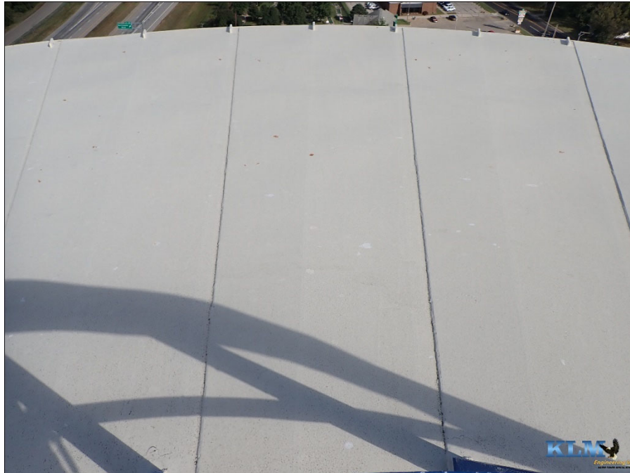
Photo No. 47 Roof coating condition
