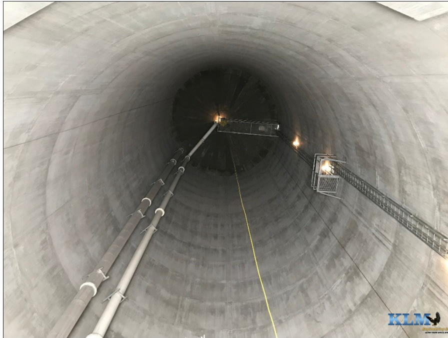
Photo No. 39 Overall condition of column interior
