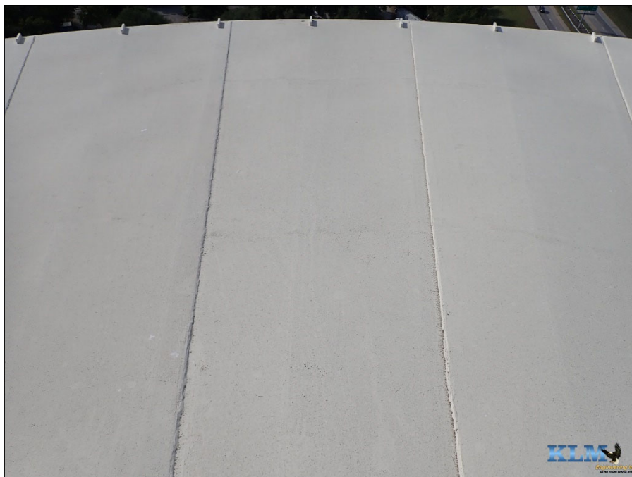
Photo No. 48 Roof coating condition
