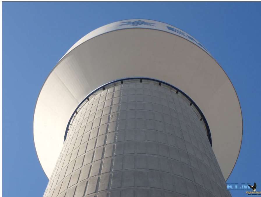
Photo No. 54 Bowl and concrete column
