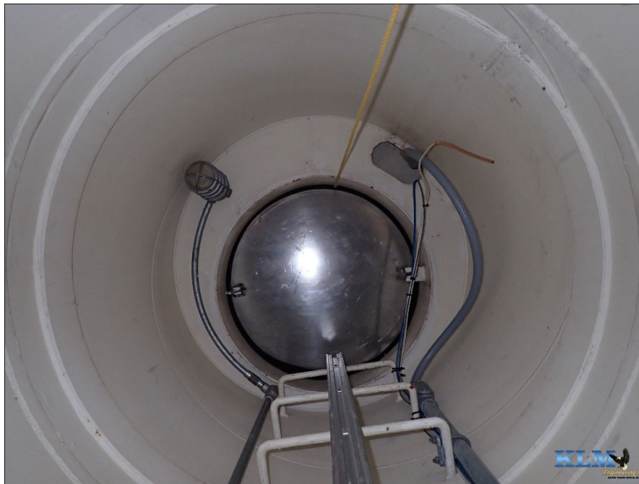
Photo No. 30 Top of drywell tube
