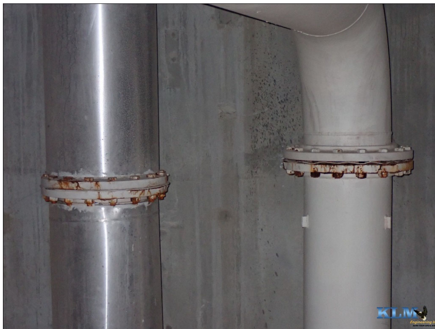
Photo No. 36 Condition of piping flanges
