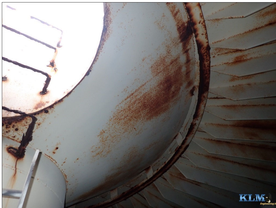
Photo No. 10 Inner cone and T-rail
