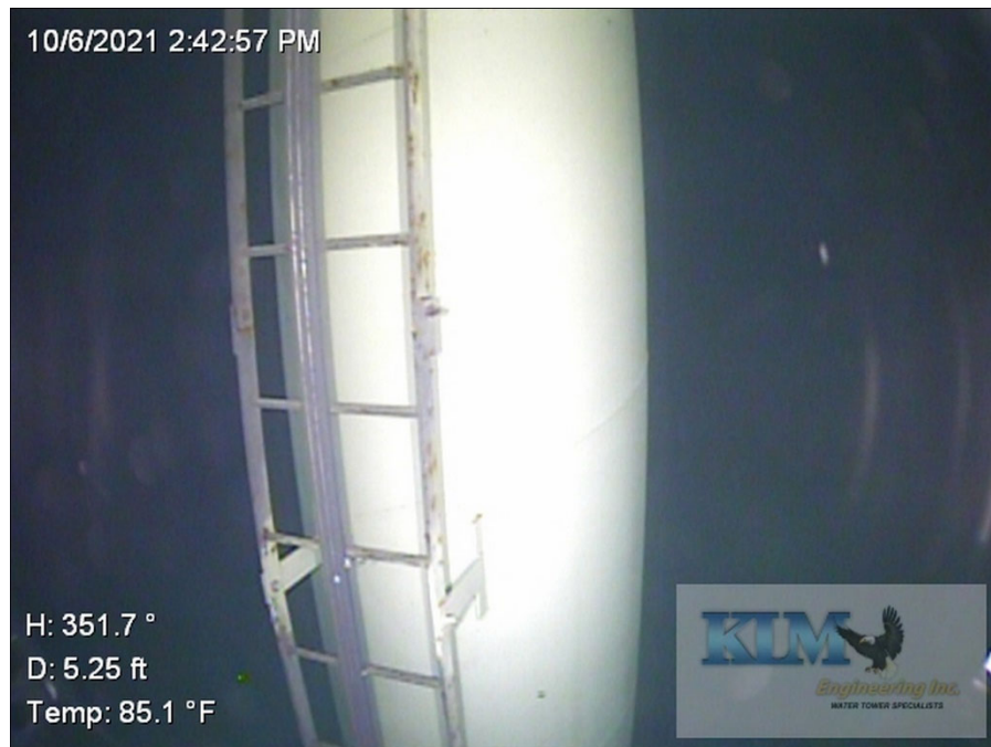
Photo No. 13 Drywell tube and ladder
