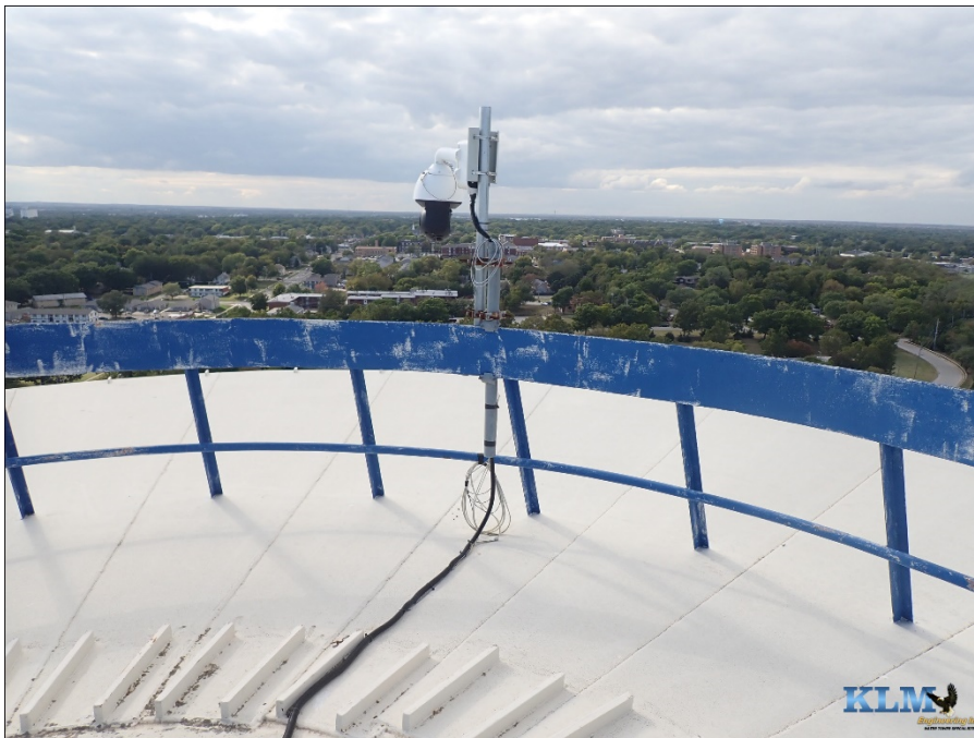
Photo No. 46 Roof handrail and equipment
