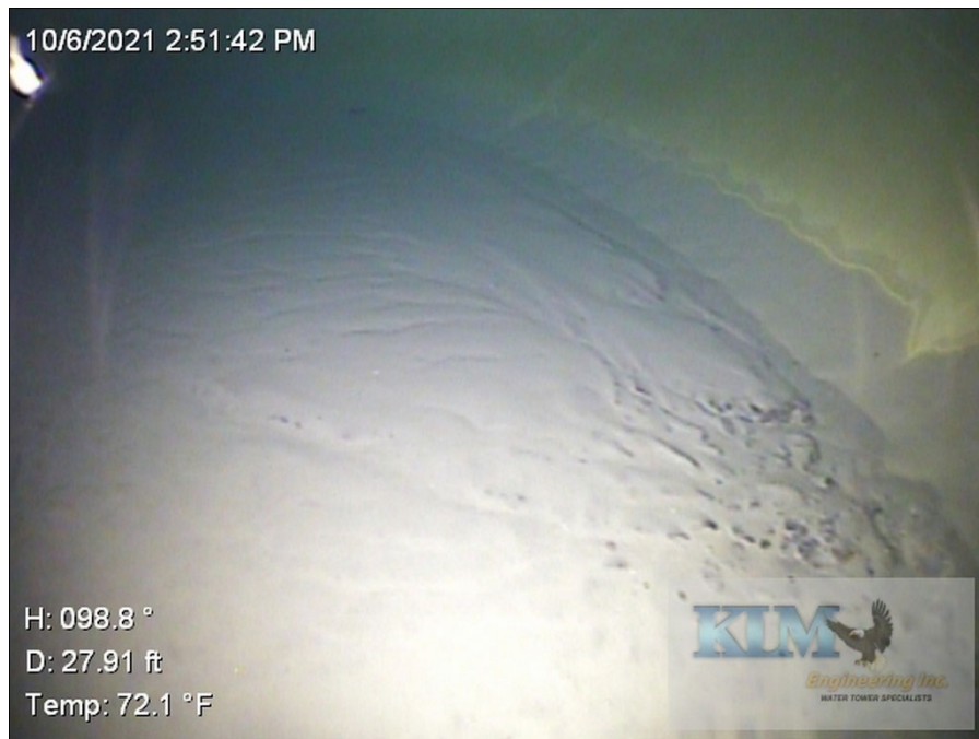
Photo No. 19 Sediment in lower bowl
