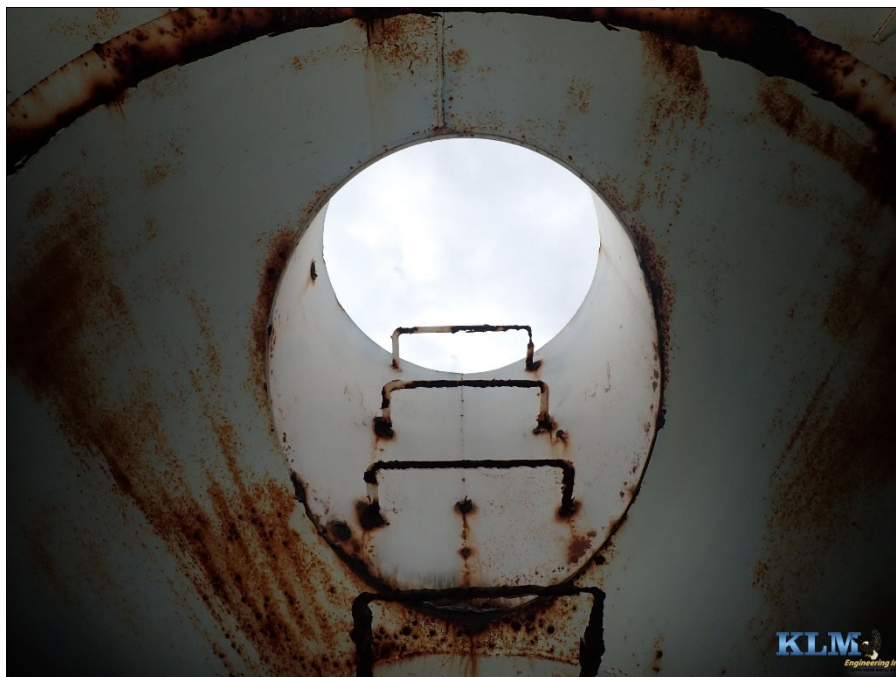
Photo No. 8 Wet access tube, Note; condition of steps
