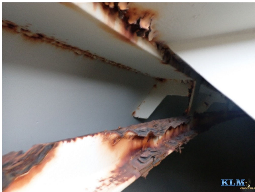
Photo No. 4 Outer T-rail and roof conditions
