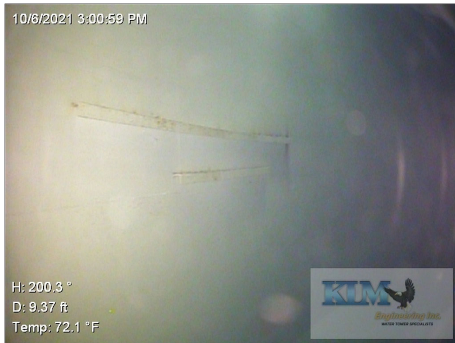
Photo No. 23 Shell condition, Note; shell erection angles
