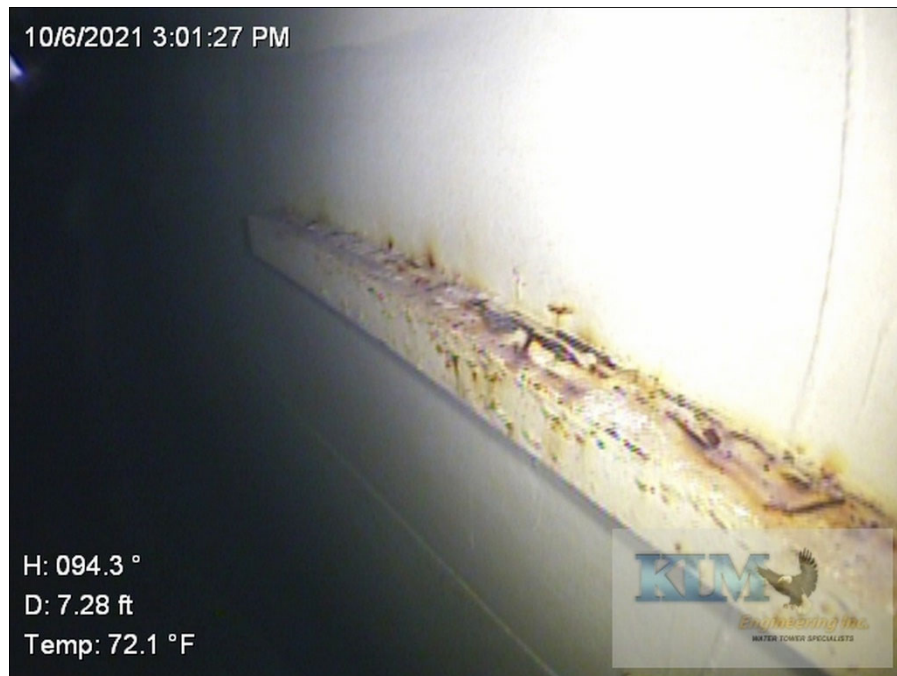
Photo No. 25 Condition of shell erection angle
