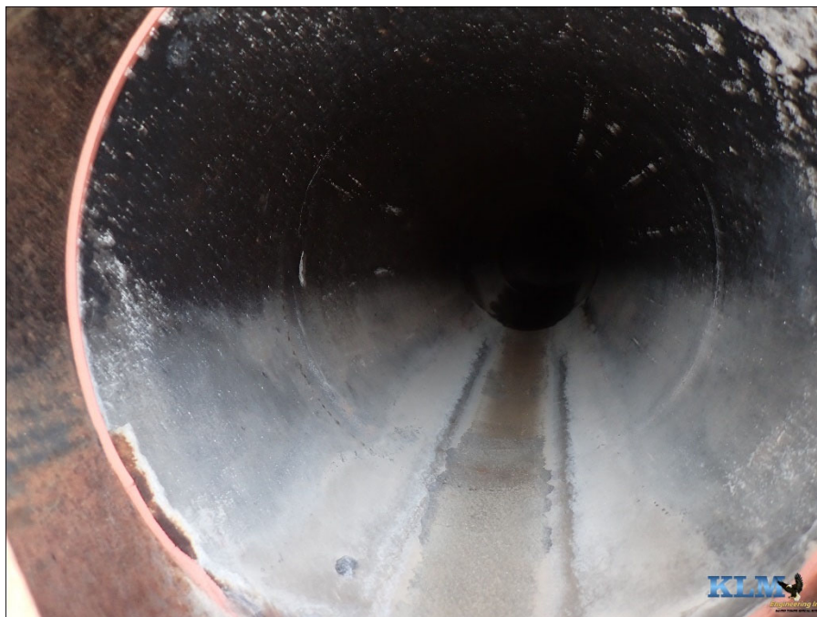
Photo No. 58 Inside of overflow pipe
